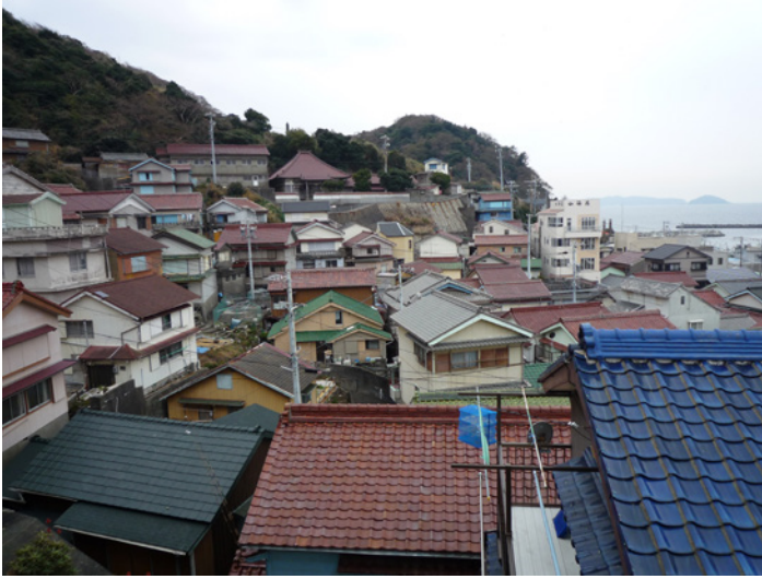
Figure 1. Rural settlement landscape of Kamishima island. The houses are mainly built in two areas: the flat land near the north coast, and on the north-west side of the main mountain slope
